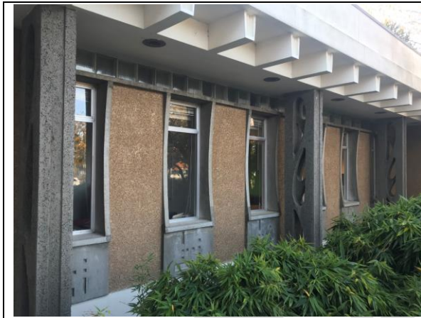
Photo 6.1 – 1963 construction. Main floor - visible original single pane windows with glass blocks (transom window) above
