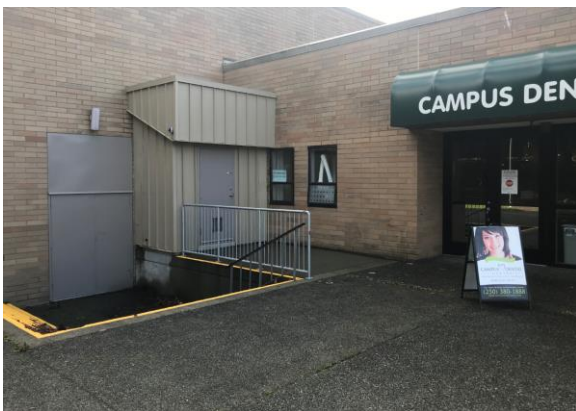
Photo 6.7 – 1974 addition. Visible pressed steel metal door, double pane punched windows and single pane storefront
