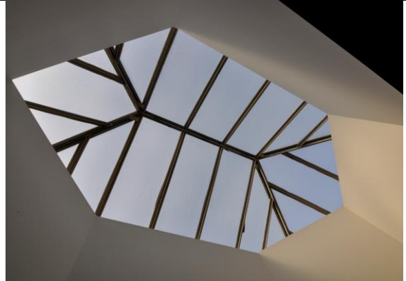
Photo 6.6 – 1963, Room B103 – Student Services Centre - visible original single pane (wired glass) in metal frame skylight.
