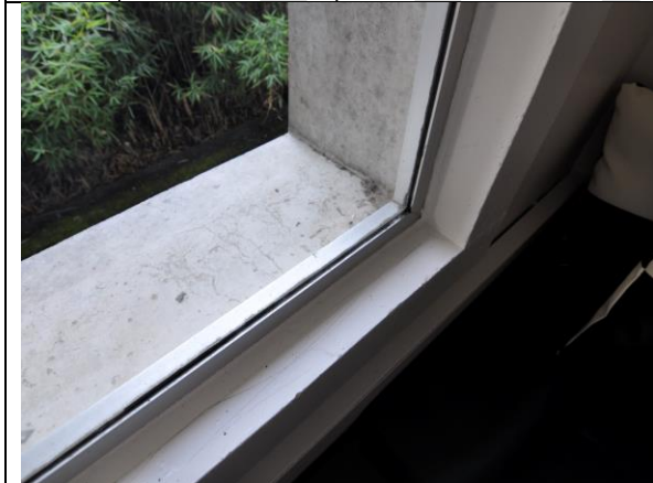
Photo 6.3 – 1963 construction. Room B107 - visible original single pane windows in solid concrete jamb.
