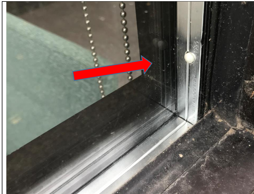
Photo 7.2 Plugs in glazing spacer indicate presence of Argon in the IGU's
