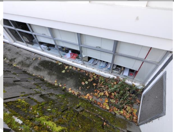
Photo 6.2 – 1963 construction. Room B011 - visible original single pane windows
