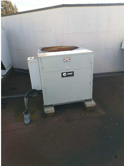
Photo 3. AHU-1 DX Unit
