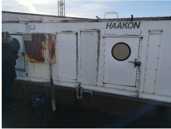
Photo 3. AHU-1 DX Unit
